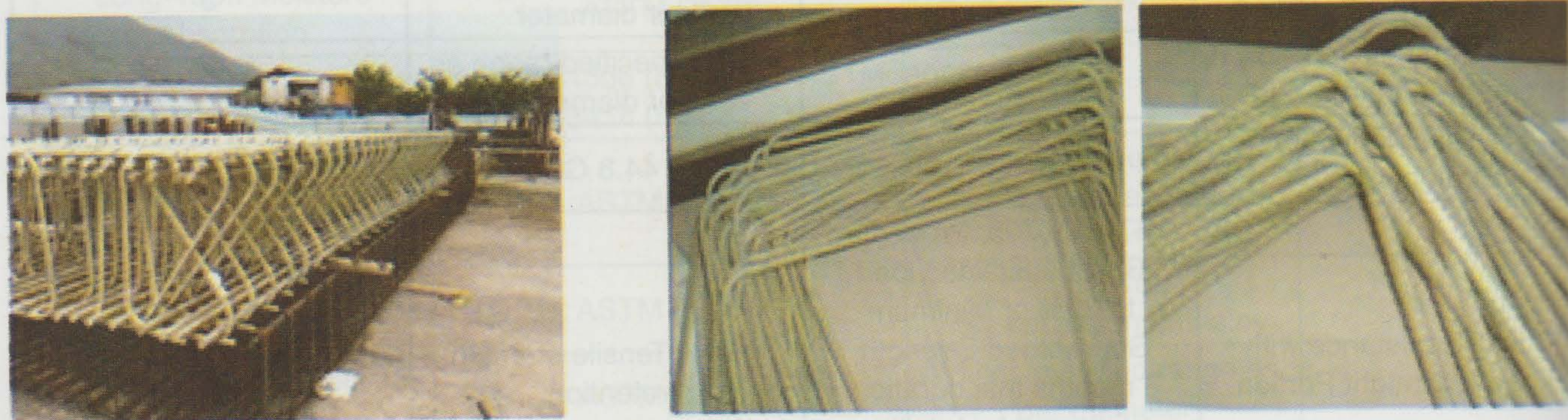
Fig. 6.1 Bending of GFRP bars ( http://www.pulwellpultrusions.com )
