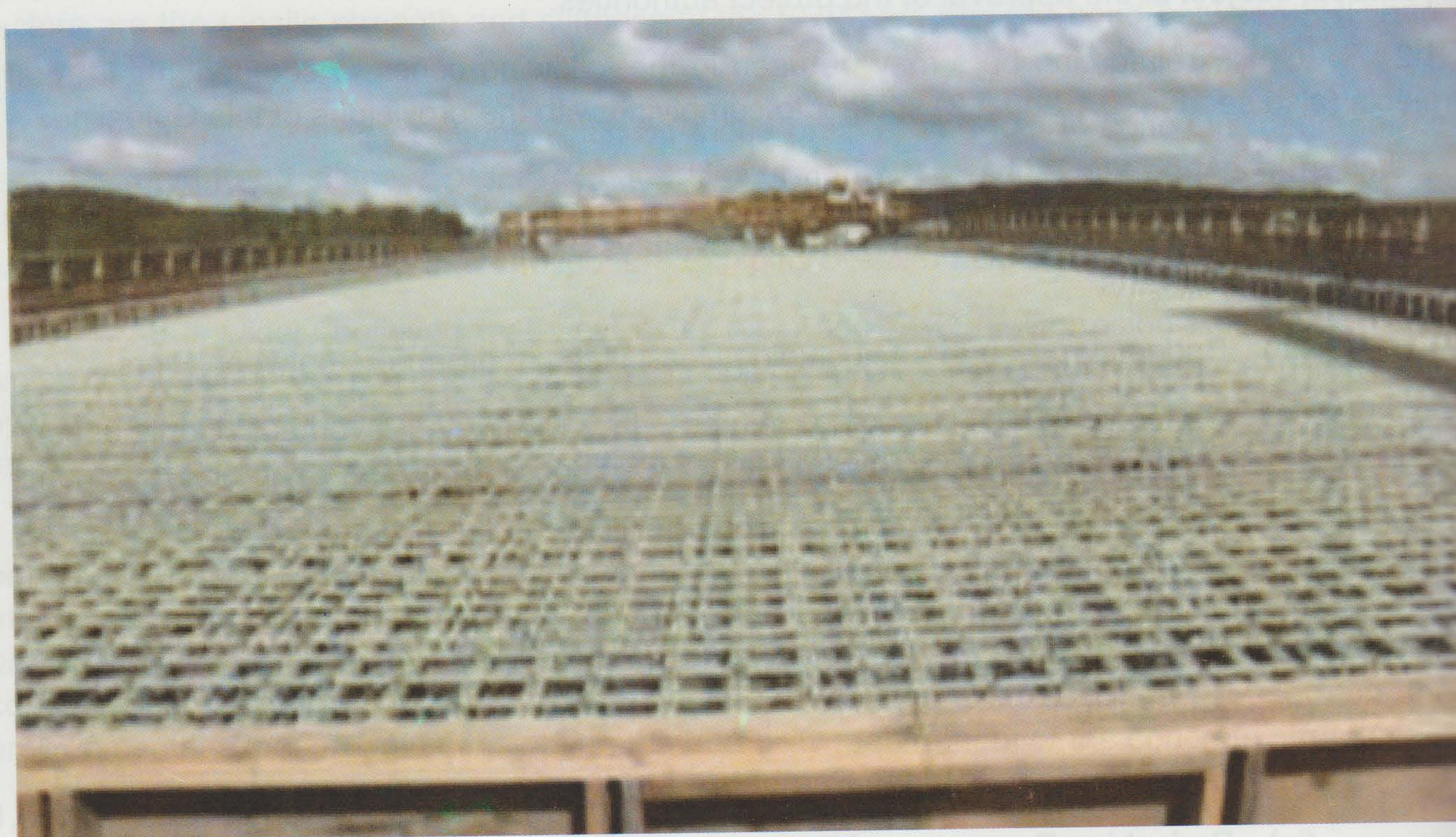
Fig. 2.2 Application of GFRP Bars in Bridge Deck Slab (Ahmed et al. 2014)
